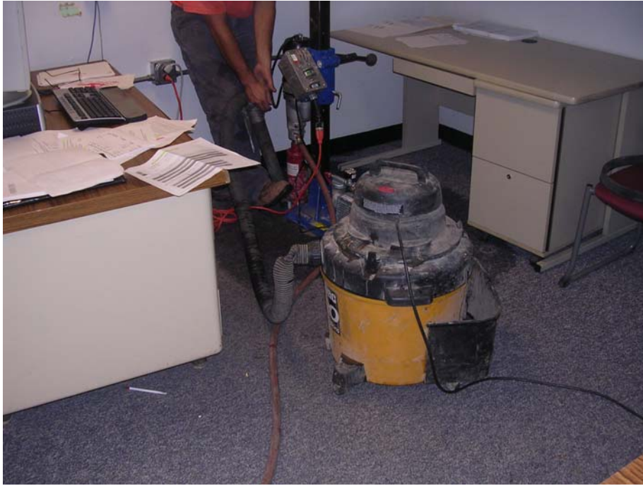
PHOTO 1 – DRILLING AT B-1 WITHIN THE EAST WING BASEMENT OF BUILDING 1.
